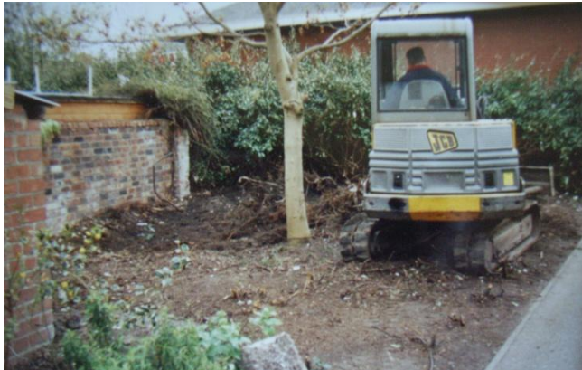
Above: a digger works on the piece of ground owned by the supermarket. Right – now a delightful courtyard garden for passers by to enjoy.
